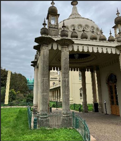
Opportunities to improve draft proofing
