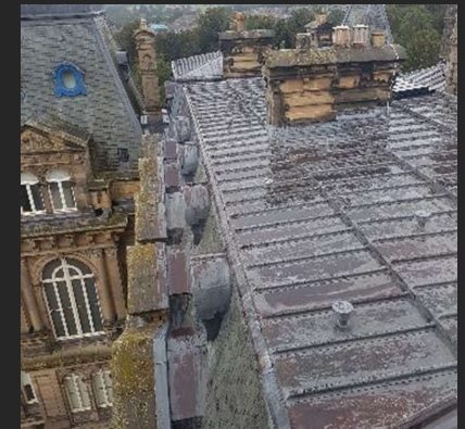
Existing flat roof with limited insulation
