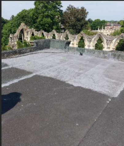
Flat roof with opportunities for PV
